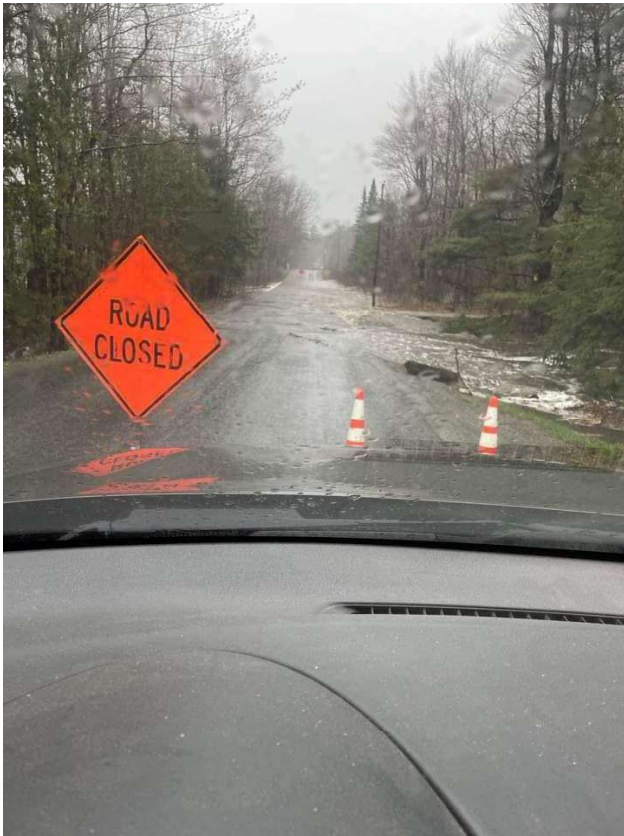
Figure 12. May 2023, Facebook Post by Geneva Asselin showing flooding on Route 143/43 Sandy River rd.
