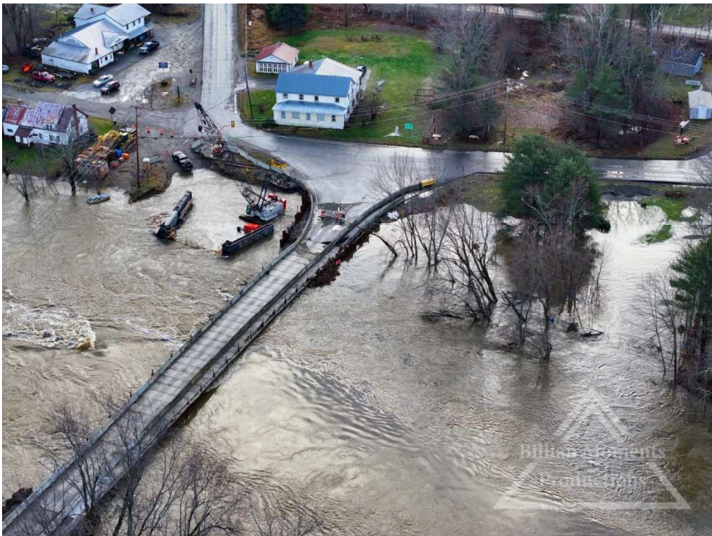
Figure 15. December 2023, Farmington Falls bridge. Photo credit to Matt Billian.
