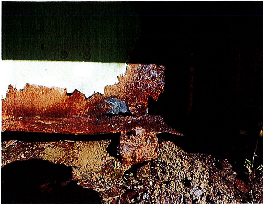
Existing beam ends, note contortion, up to 100% section loss, damage is typical all beam ends
