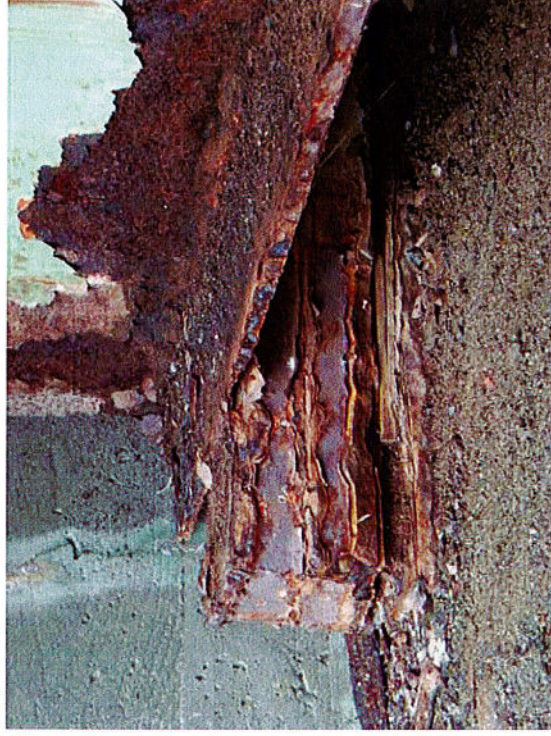
Photo 5: Section loss at beam end (Typical)
