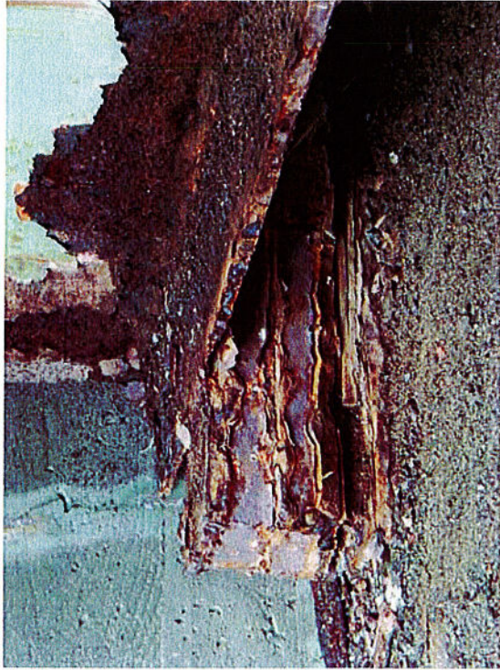
Photo 5: Section loss at beam end (Typical)
