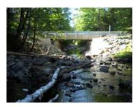
Greg performed final structural design of two bridges which are innovatively mildly reinforced inverted precast concrete t-beam structures in Starks, Maine in 2013 & 2014. The photo to the left is of West Mills Road over Lemon stream, which was value engineered and existing abutments salvaged. The second structure is the Mayhew road over Pelton Brook, which necessitated a realignment and had integral abutments founded on drilled well casings.
