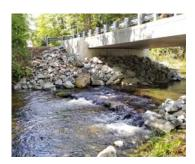
Preliminary & Final Design of Tannery Brook Bridge on Dority Farm Road in Mariaville, ME. This project was designed and completed with only a 14 day road closure to minimize the impact on the residents living beyond the bridge. Precast abutments, wing walls, and superstructure designed to accelerate construction to allow this shortened closure. 2016 through 2018
